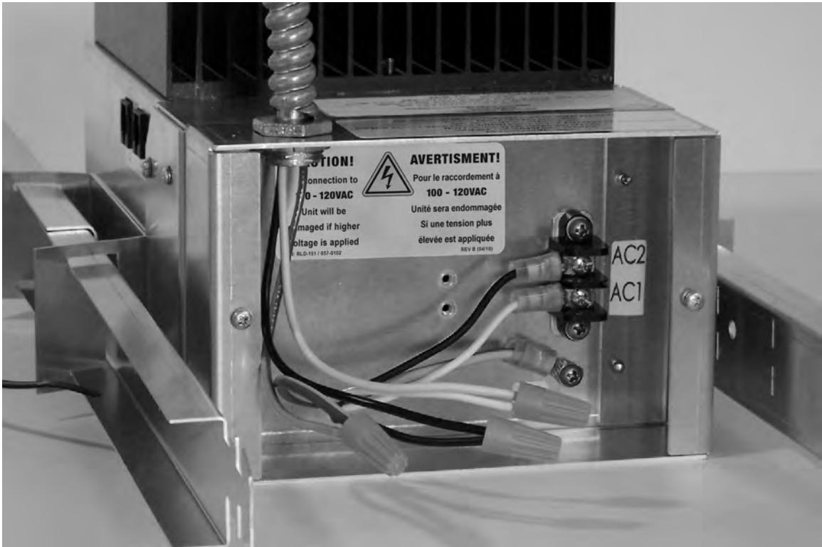
Figure 10: Completed Wiring in Junction Box
